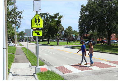
Improved pedestrian safety
